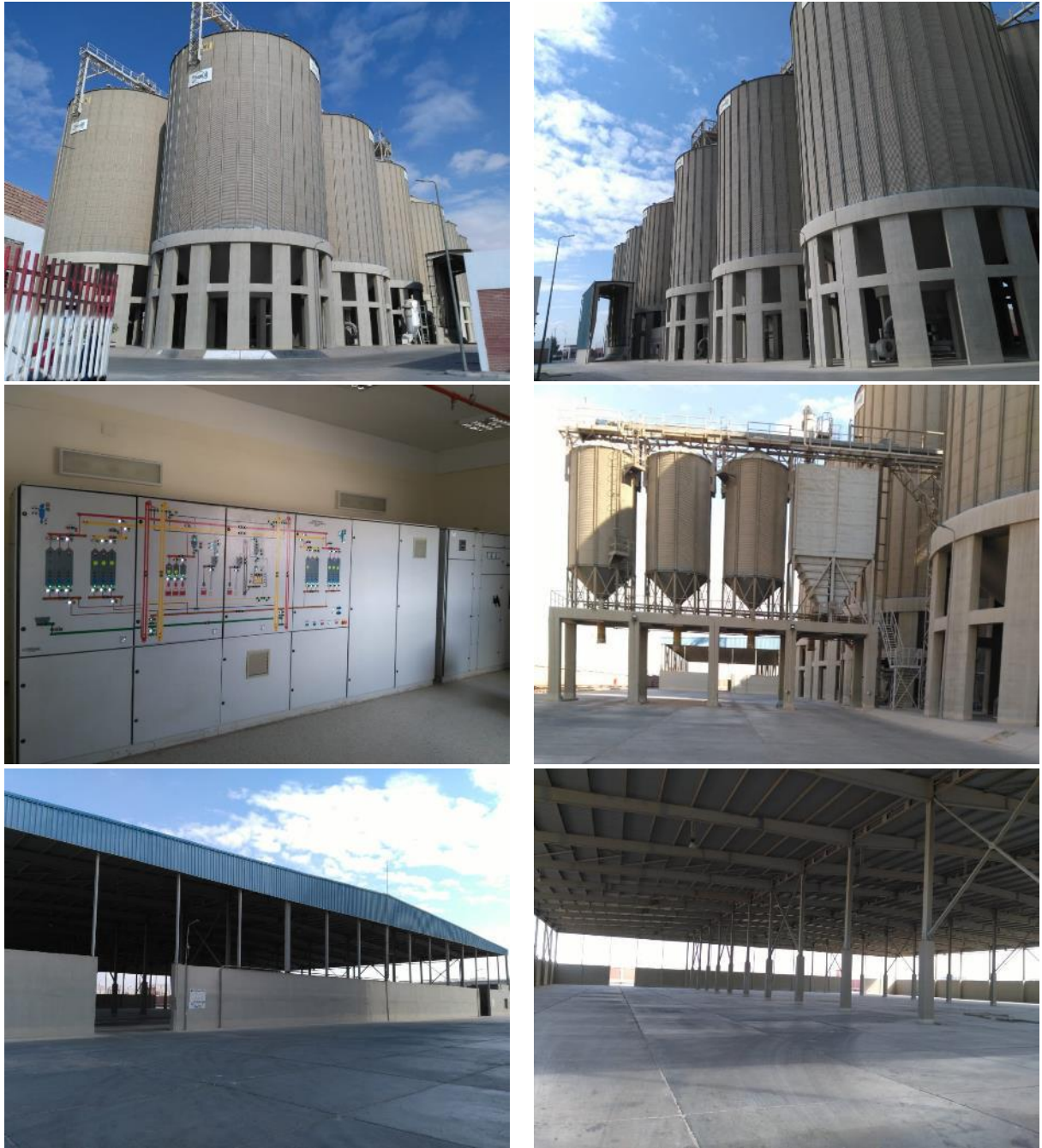
Figure (V.3): Some photos from Assuit Silo Complex.
